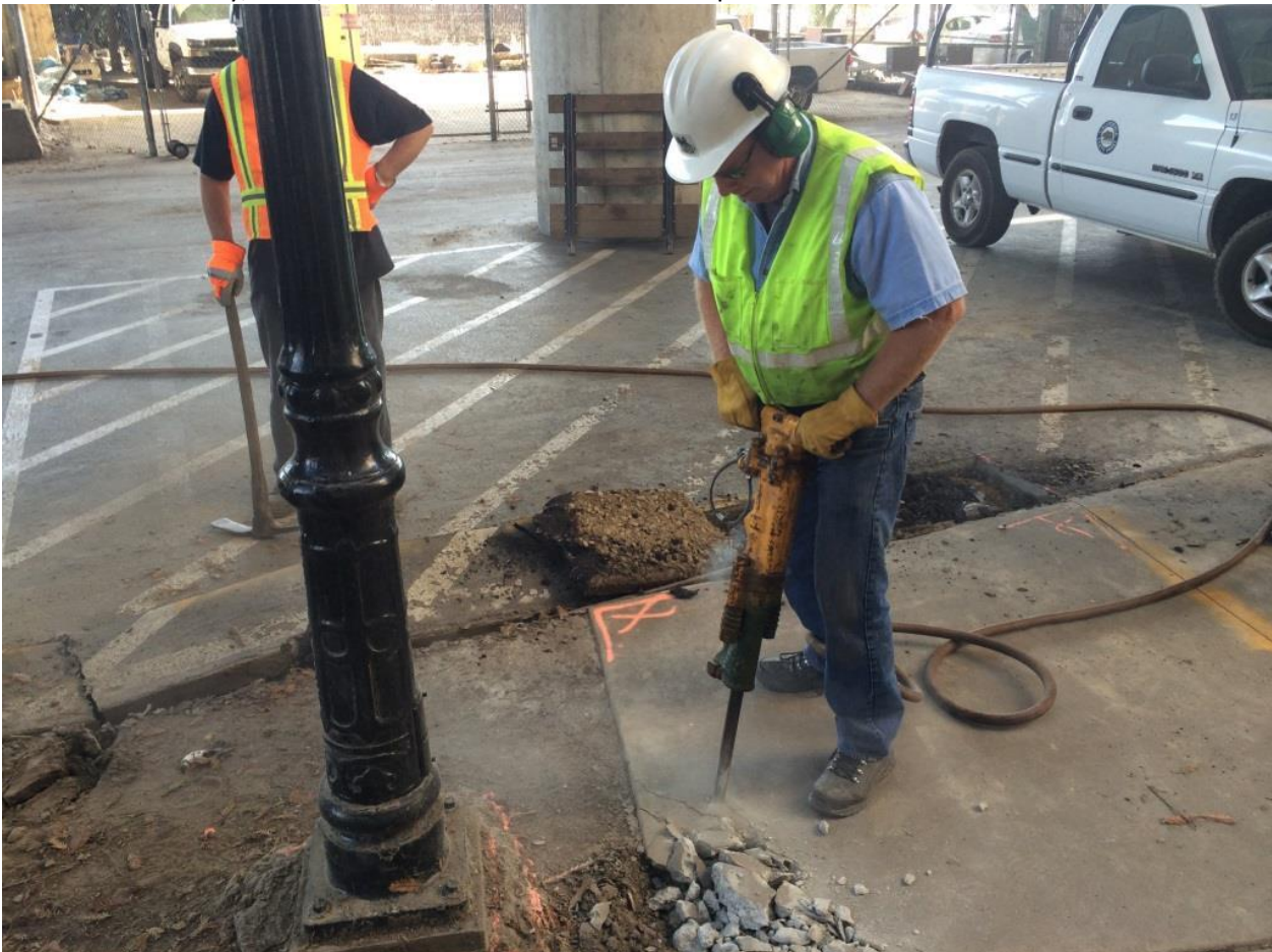
Ed got the ball rolling with the first jackhammering of the day
