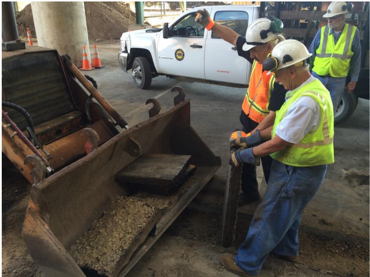
Fred and Clem loading asphalt chunks into the bucket of the back-hoe
