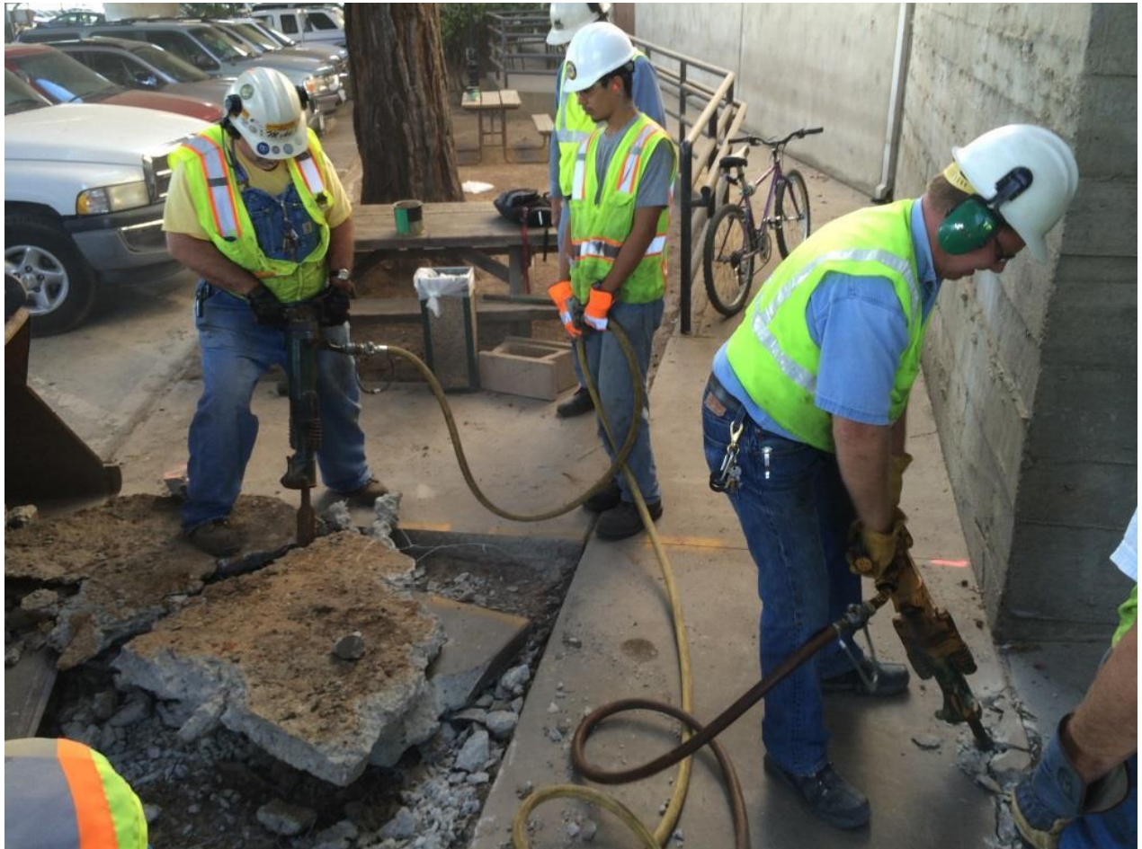
Mike F. and Ed jackhammer away
