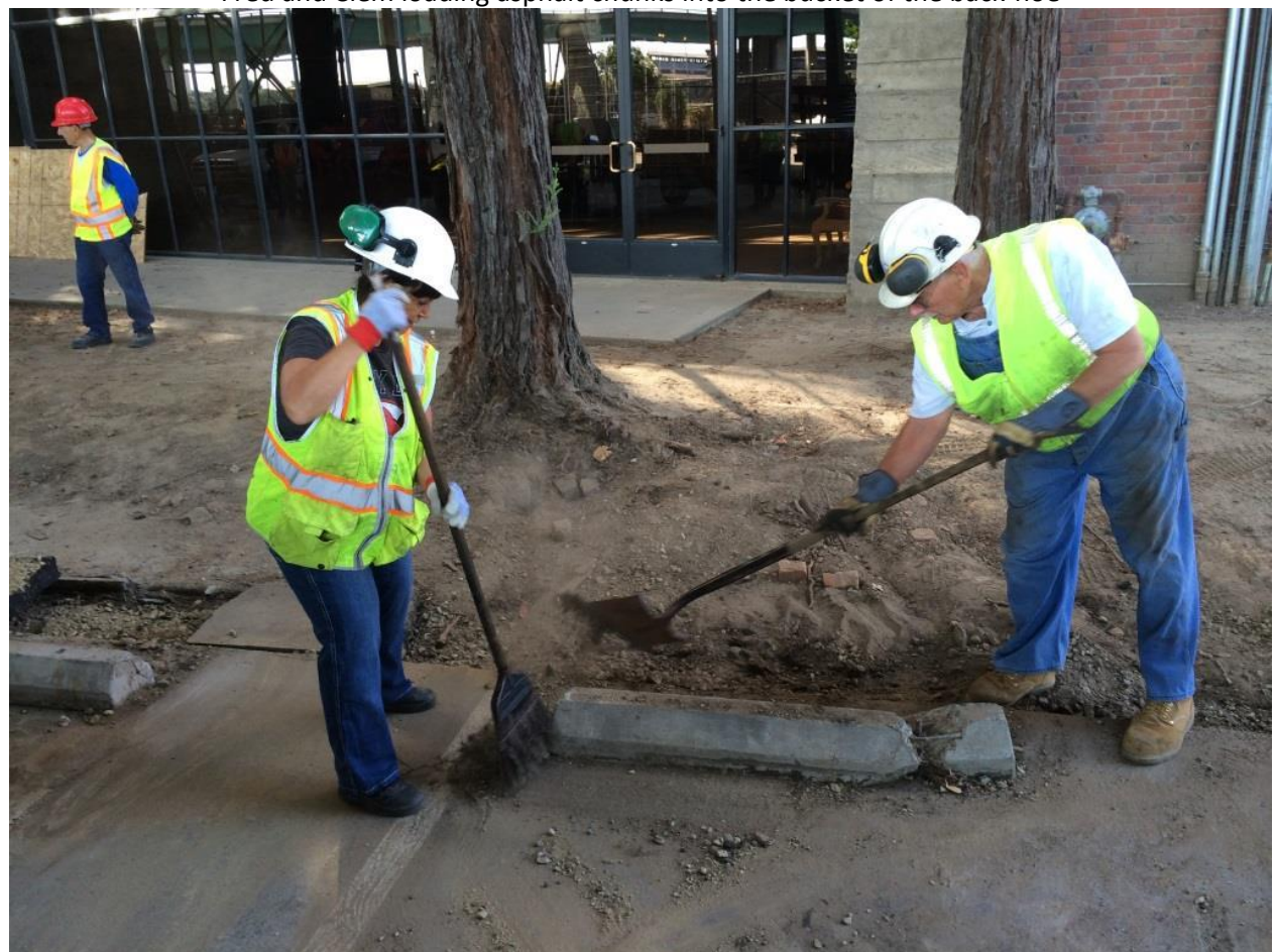
Pam and Clem start removing the debris
